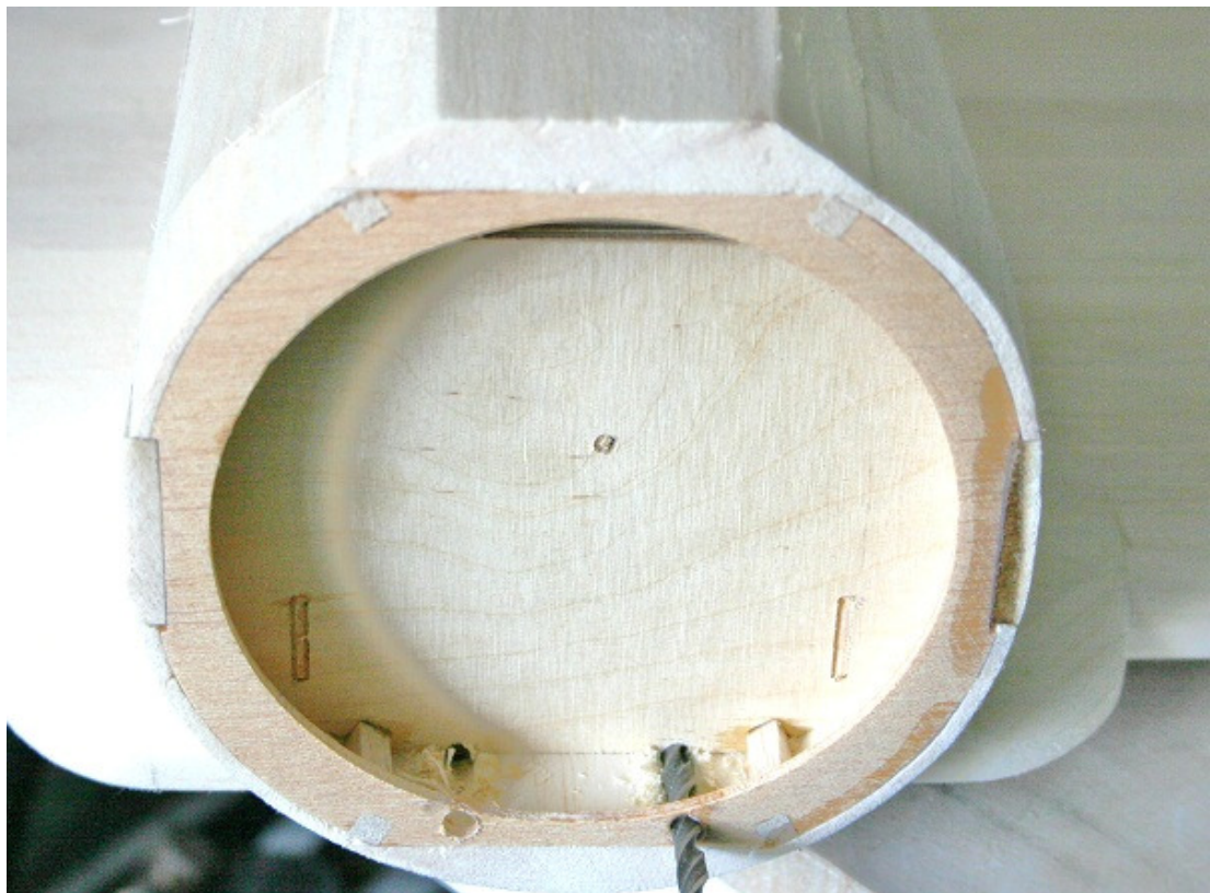
Drill through into wings for wing dowels
